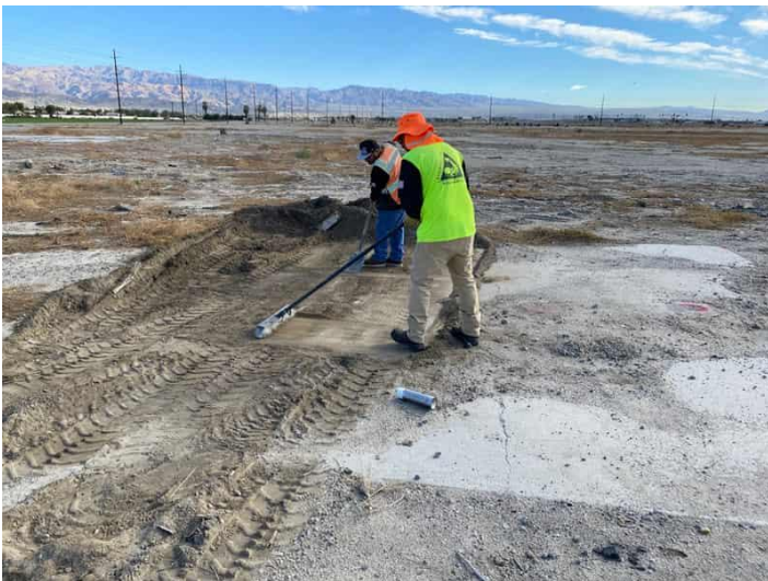
Photo Description | Anomaly Site Pre-Excavation Activities
